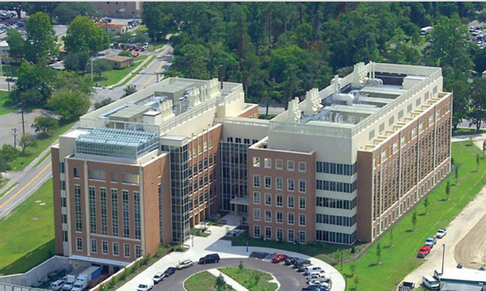
University of Florida - Genetics Institute & Cancer Research Center Generator Stack & Boiler Stack
