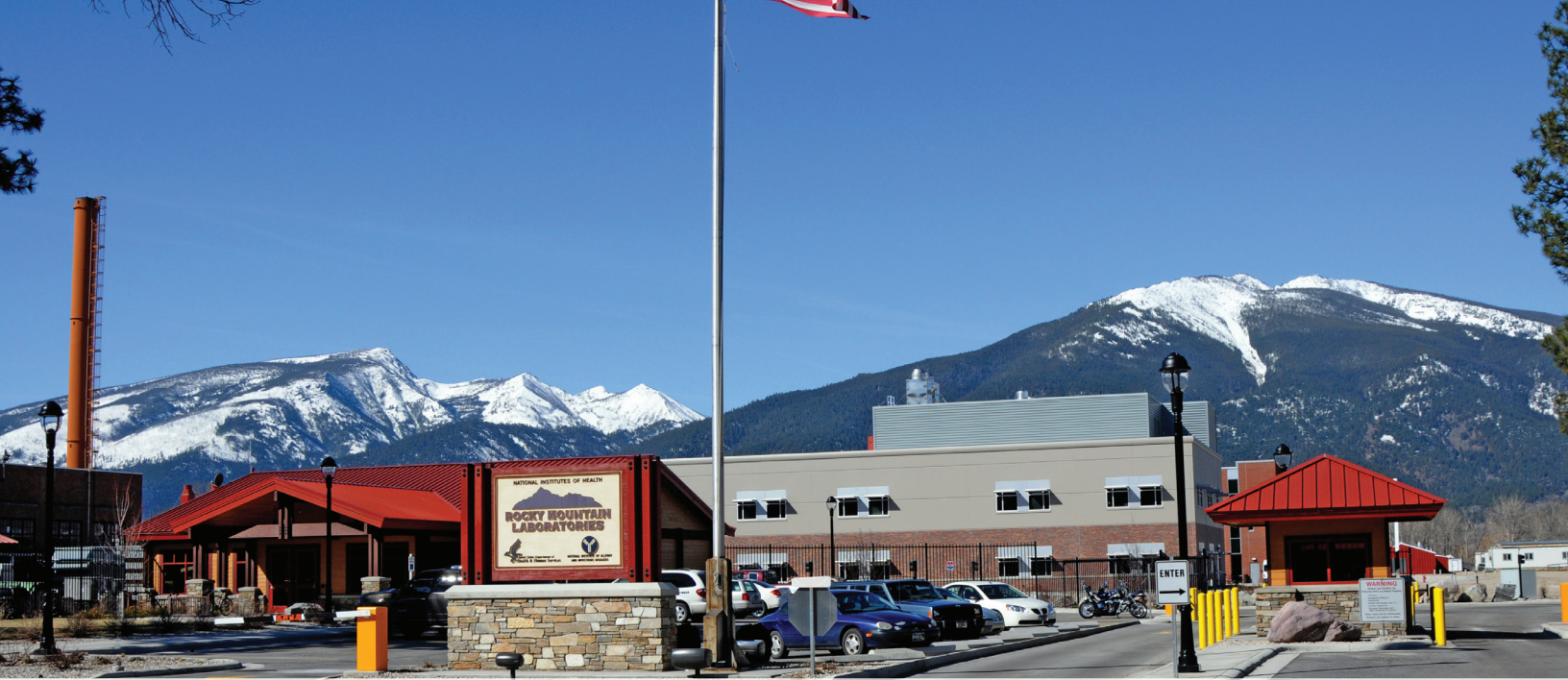
Rocky Mountain Laboratories Freestanding Stack
