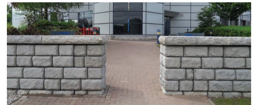
Build Barrier and Force Protection Walls
