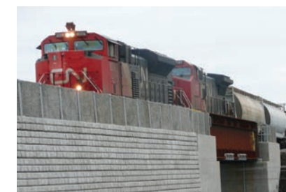
Handling Live Loads
